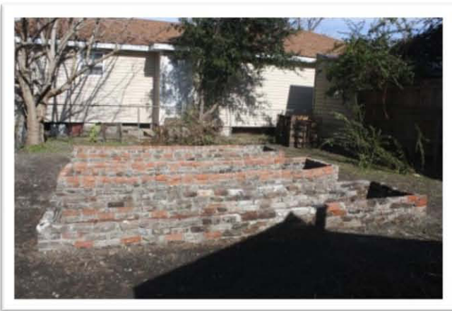
February 2010 Raised beds constructed
