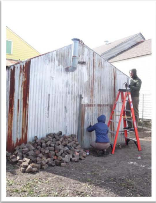
January 2010 Shed repair and redesign
