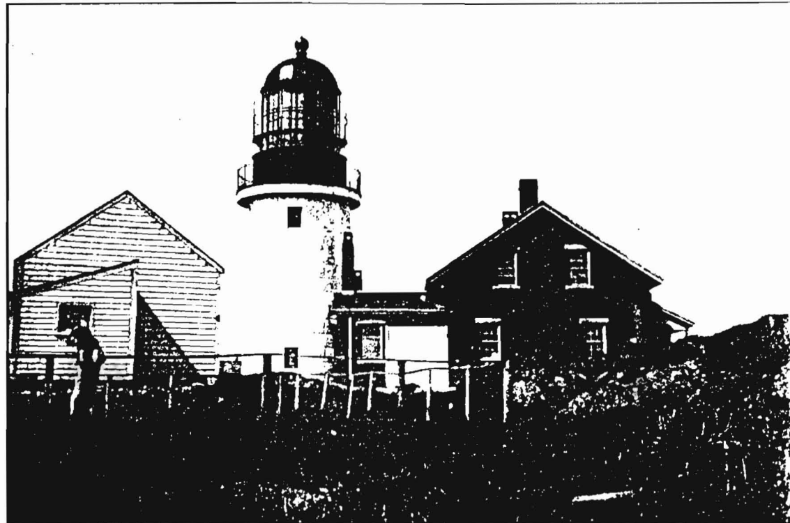
The Seguin Island lighthouse as it appeared in 1904. (Photo by Capt. Jim Perkins, courtesy of Friends of Seguin Island)
