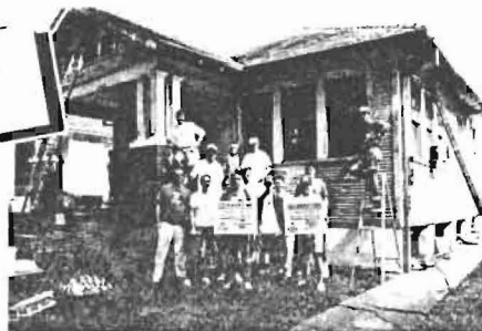
Deusch, Kerrigan & Stiles/IBM Corporation: 4631 Banks
