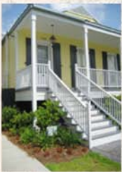
A Successful Elevation Project
