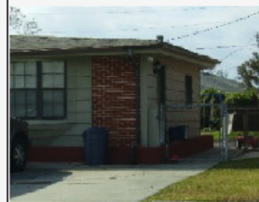
This homeowner built a small floodwall surrounding the structure
