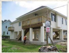
Elevation Work Nearing Completion
