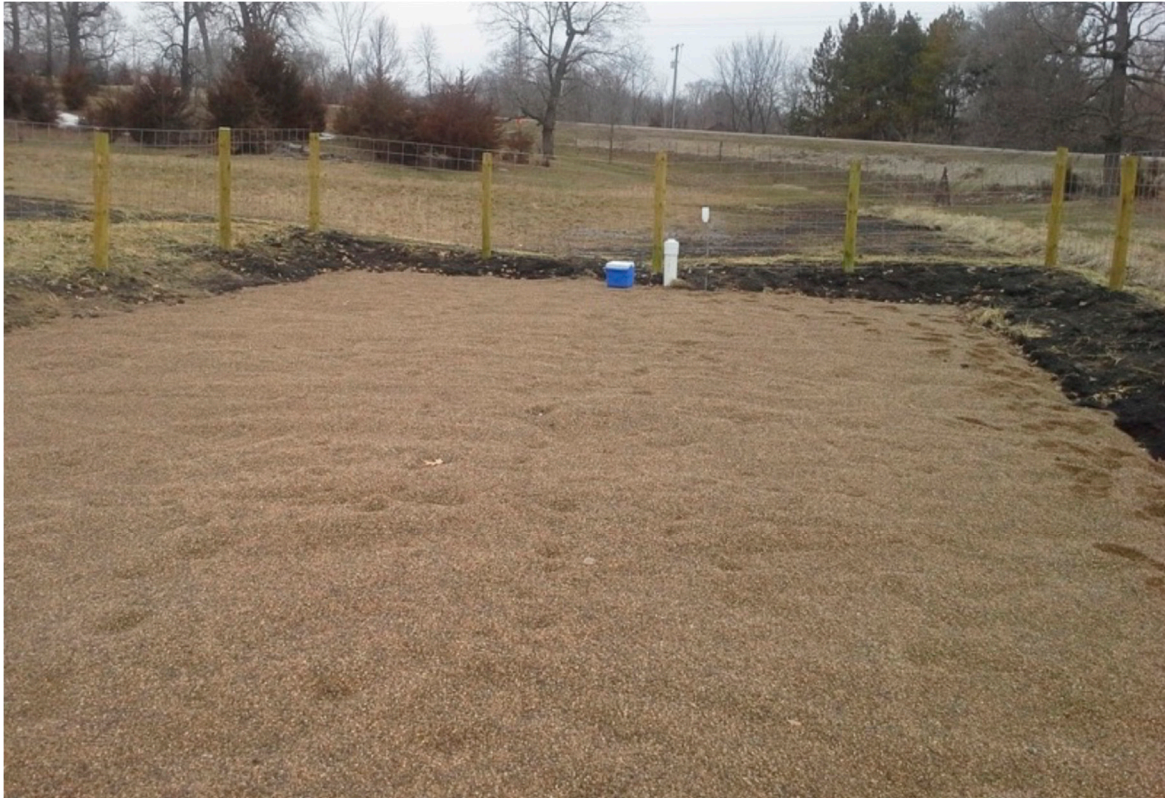
Figure 1. Site photo of Iron Enhanced Sand Filter (IESF) shortly after construction.
