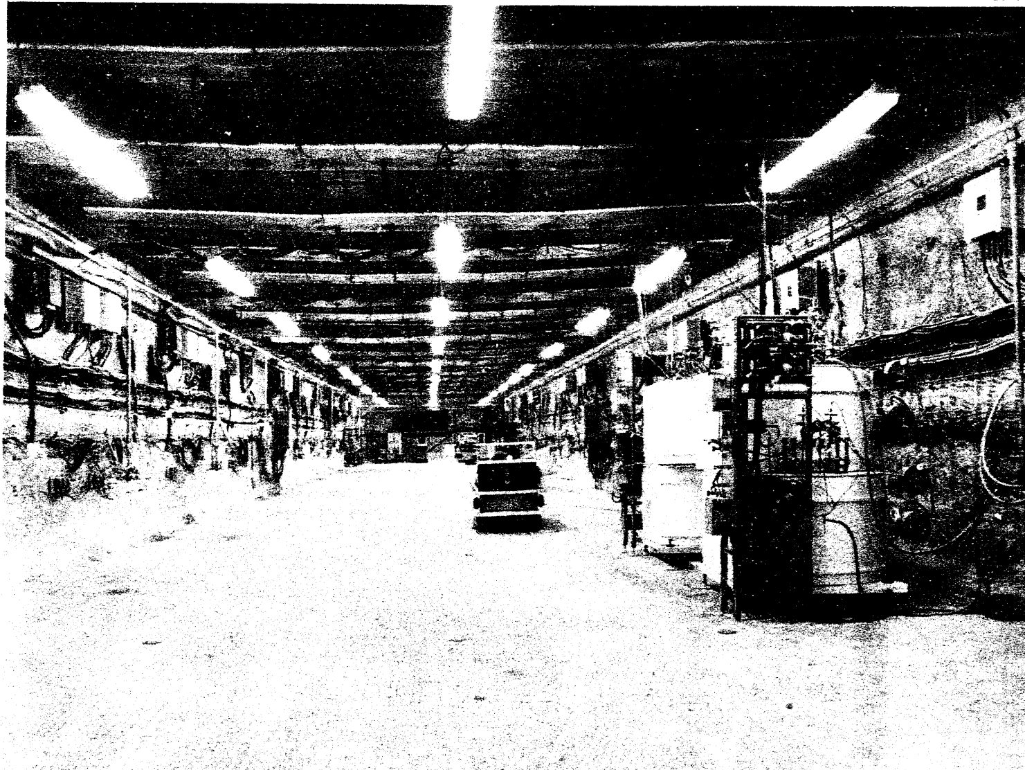
Empty transuranic waste test containers (bins) located in an underground Waste Isolation Pilot Plant (WIPP) waste storage area where tests are being planned to demonstrate that the WIPP facility will suitably hold wastes for disposal and meet regulatory requirements. (Courtesy of Westinghouse Electric Corporation, WIPP Project Office, Carlsbad, New Mexico, and MAC Technical Services Company, Albuquerque, New Mexico.)
