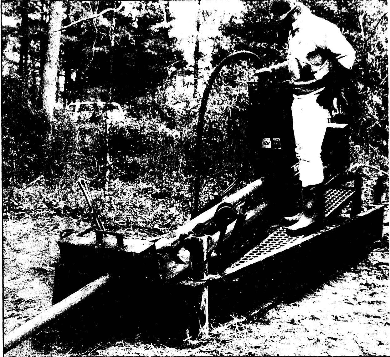
Figure 3. Ditch Witch True Trac drill rig.
