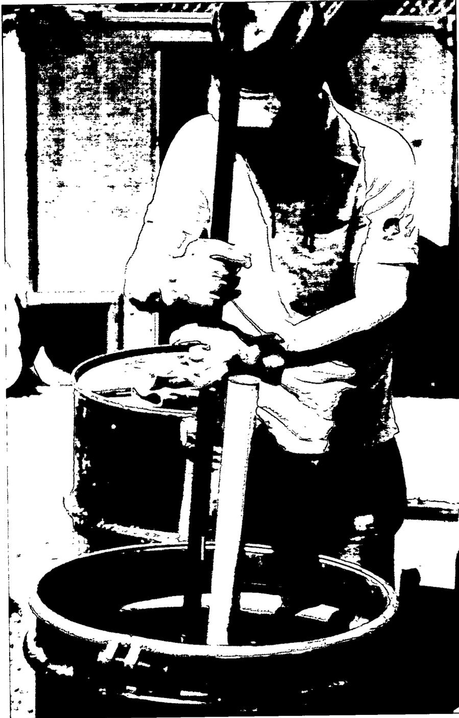
Fig. 8. Packing the crushed tuff (known water content) to a known bulk density in a 15-cm lift in a calibration drum in the 1982 calibration study.
