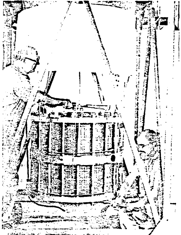
Fig. 4. 8 T background coil fully assembled.
