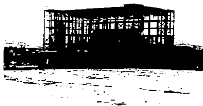
FIG. 1. MFTF building during construction in the early 1950's.
