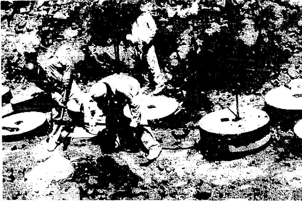
Fig. 2. Breaking the seal on the cask lid.
