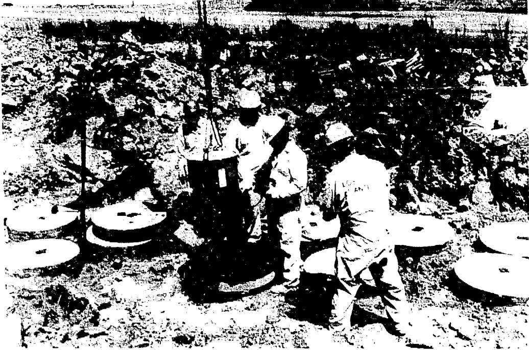
Fig. 4. The drum is removed from the cask, monitored, examined, and photographed.
