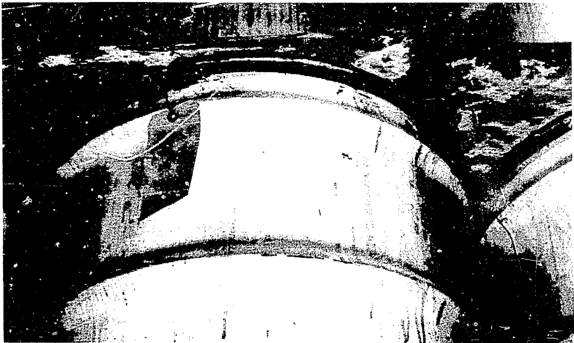
Fig. 11. Drums adjacent to shaft, coated with rust inhibitor Texaco CPD L. Note fire-retardant bleeding out of plywood.
