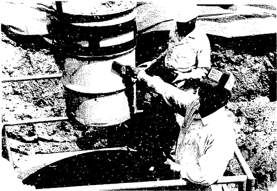
Fig. 12. Uncoated ^{239}\text{Pu} -contaminated waste drum being retrieved from bottom of shaft, Cell 2.
