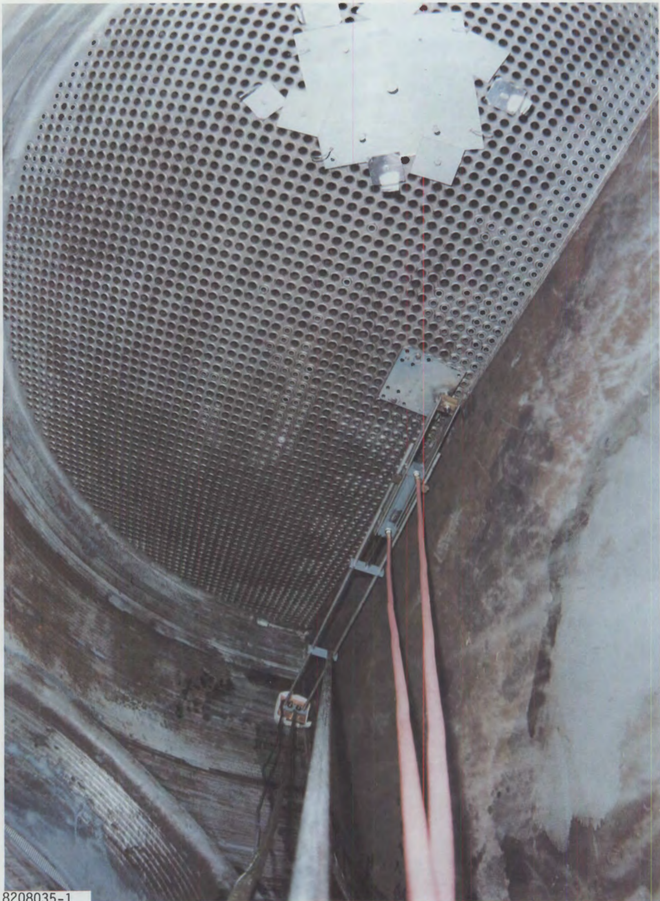
FIGURE 4-14. Electropolished Area on the Inconel 600 Divider Plate
