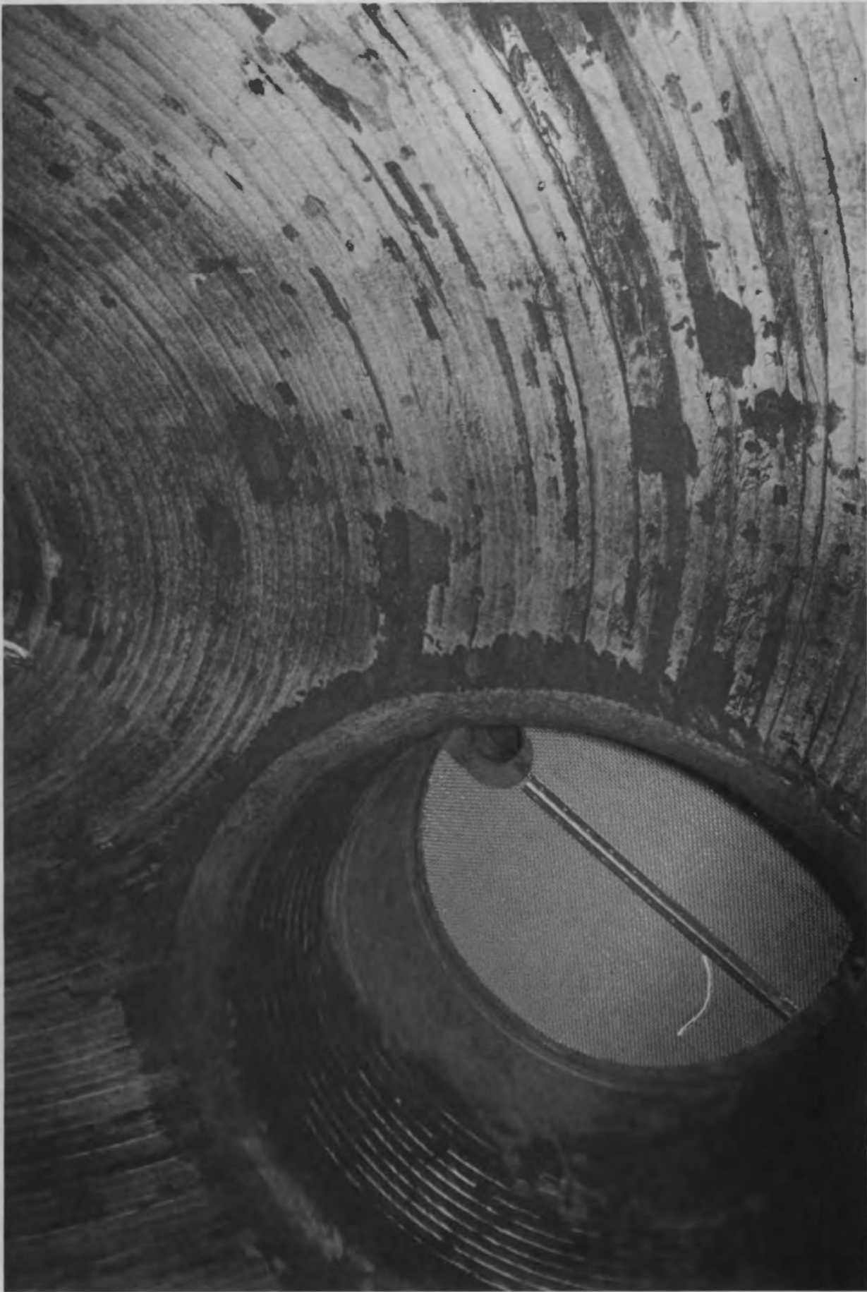
FIGURE 2-12. Installed Nozzle Cover Coating and Hold-Down
