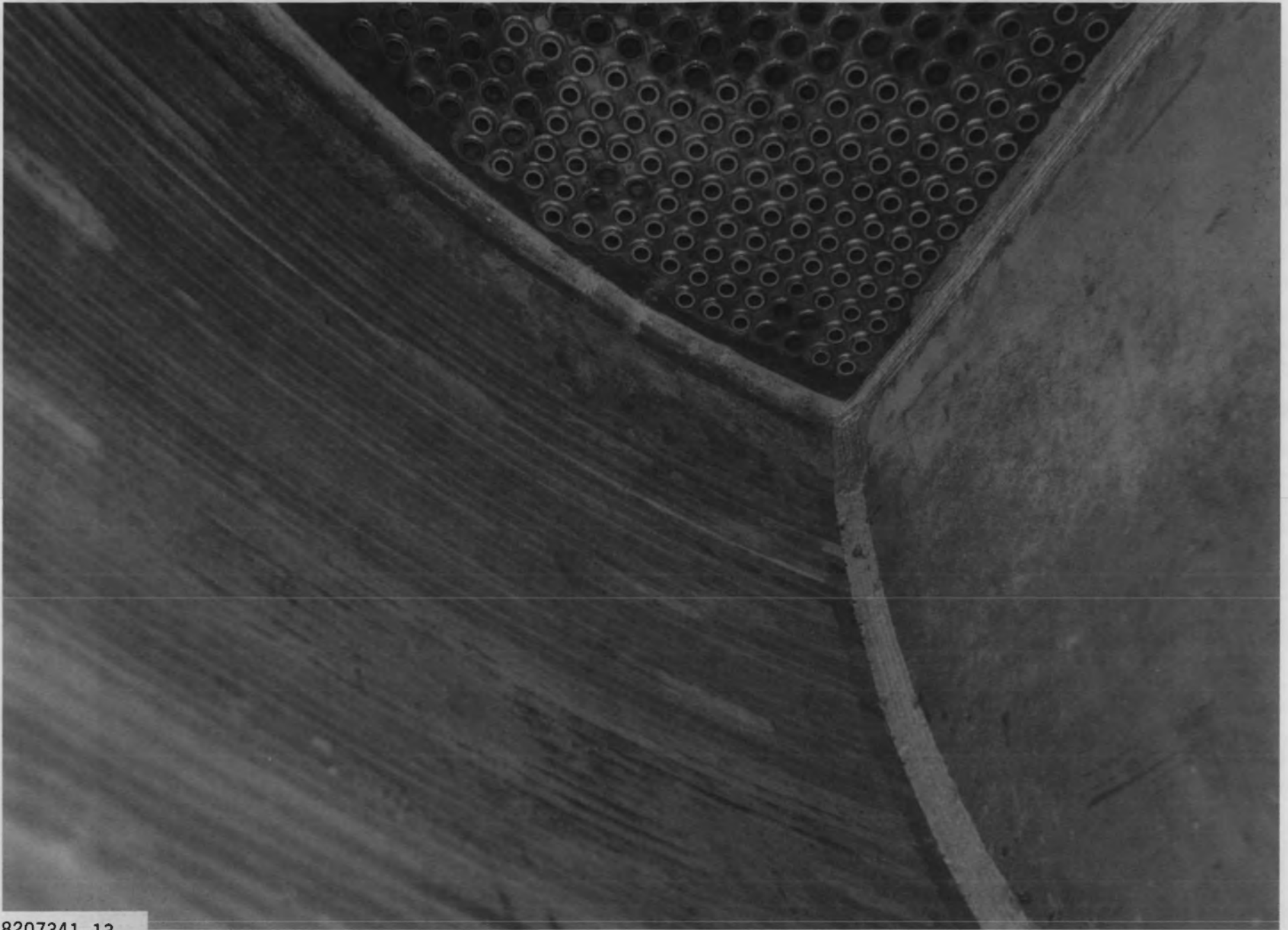
FIGURE 3-17. Cold Leg Surfaces After High-Pressure Water Rinse
