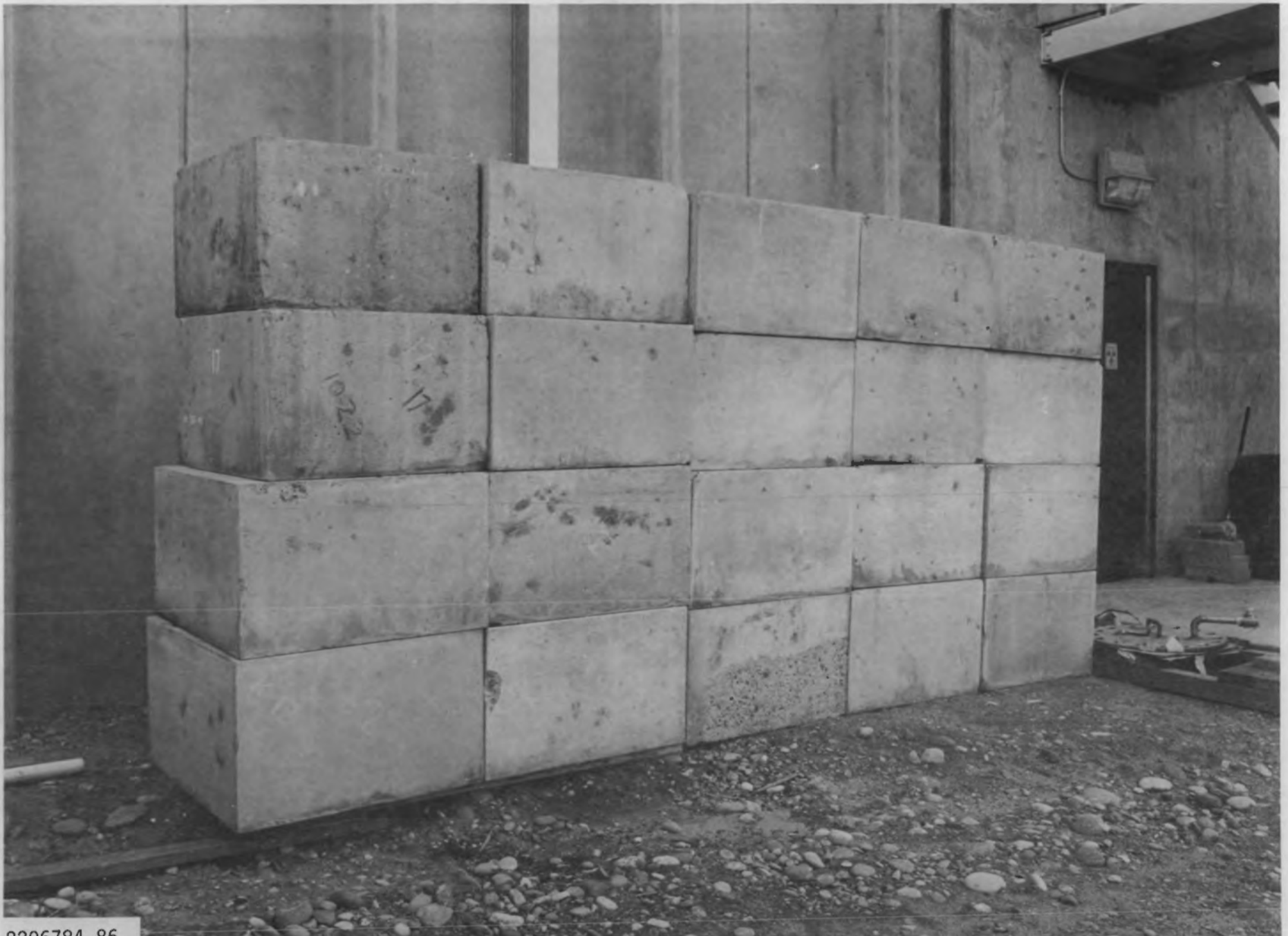
FIGURE 2-8. Concrete Block Shielding Wall Outside the Steam Generator Examination Facility
