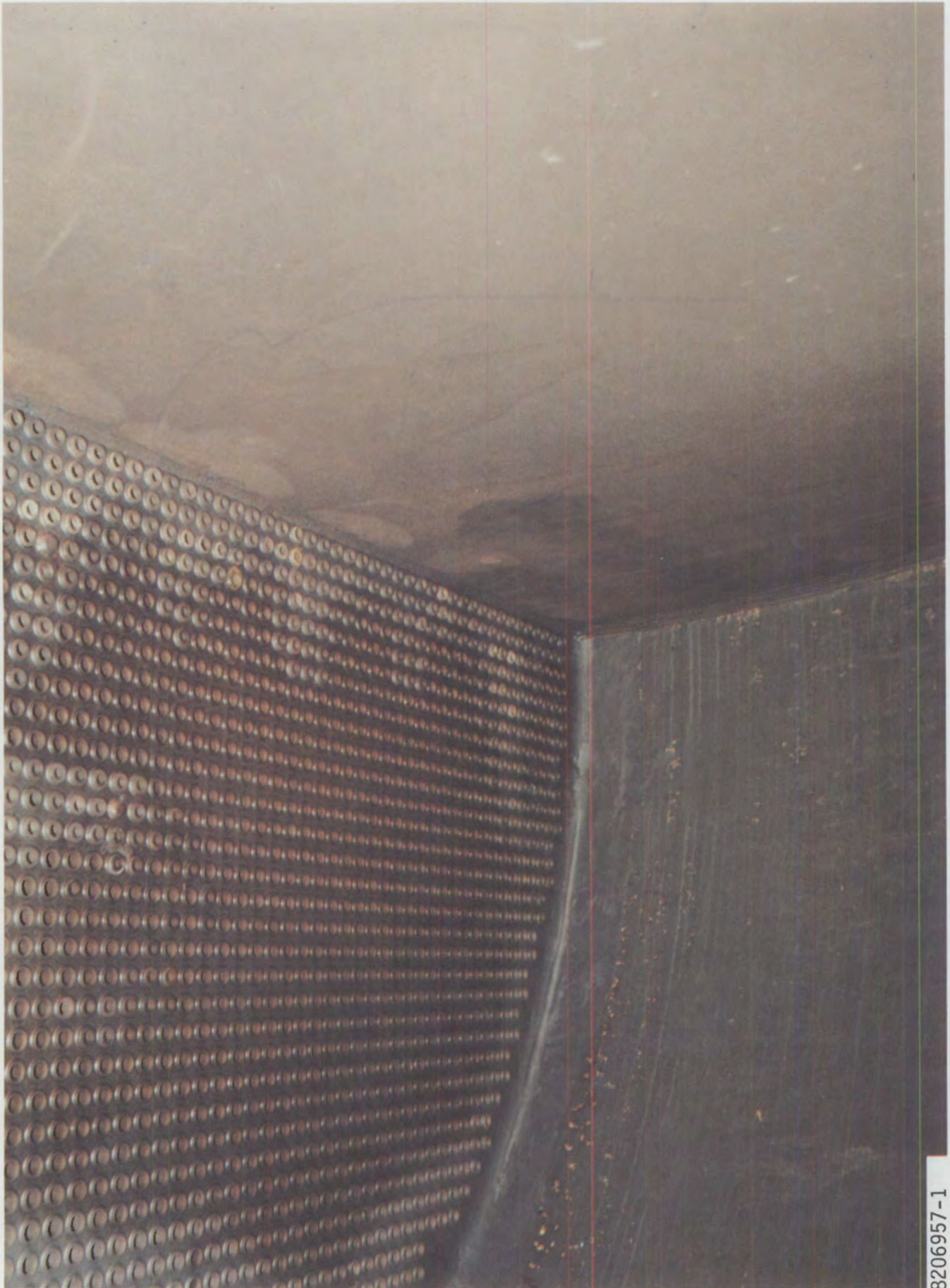
FIGURE 4-10. Hot Leg Surfaces Before Decontamination
