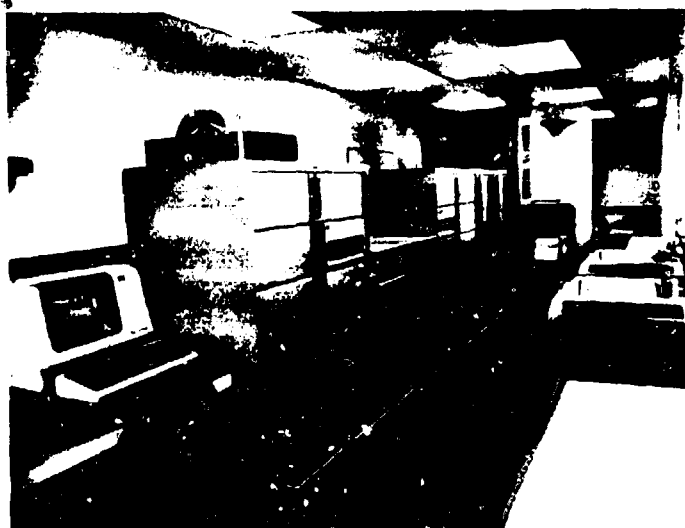
Fig. 1. FPA Control Room.
