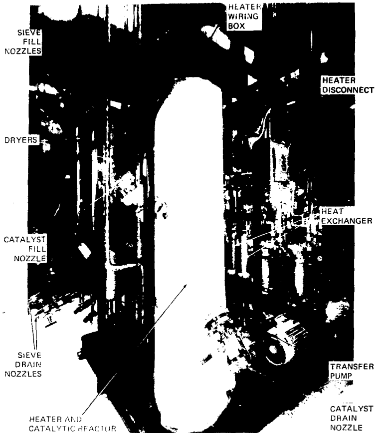
Figure 15 VERS skid final configuration.
