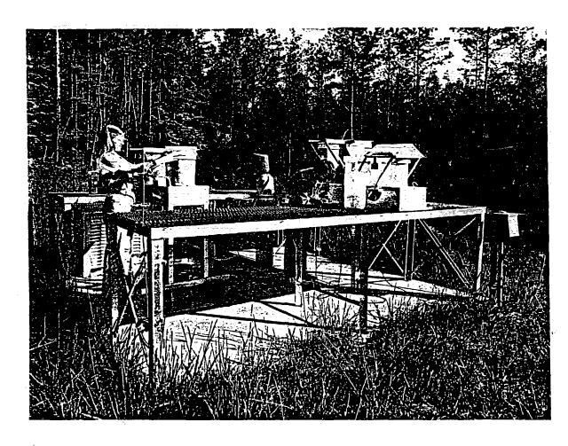
Figure 2. Apparatus for collection of precipitation as wetfall-only, shown for comparison with dry collectors. These devices are situated in forest clearings, as illustrated, and beneath different canopy types. Wetness sensing grids are used to automatically expose sealed collectors to wet deposition.
