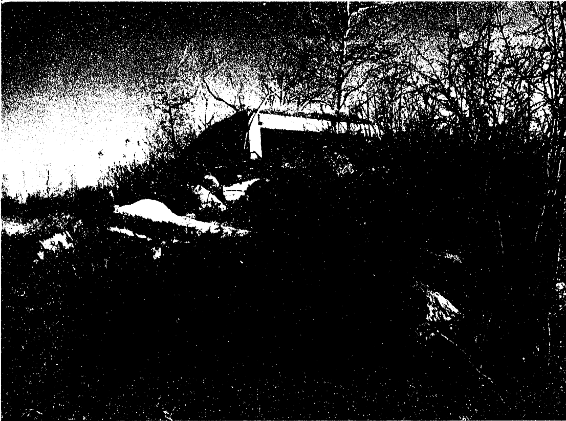
Fig. 10. View of the concrete bunker prior to its excavation, looking northeast.
