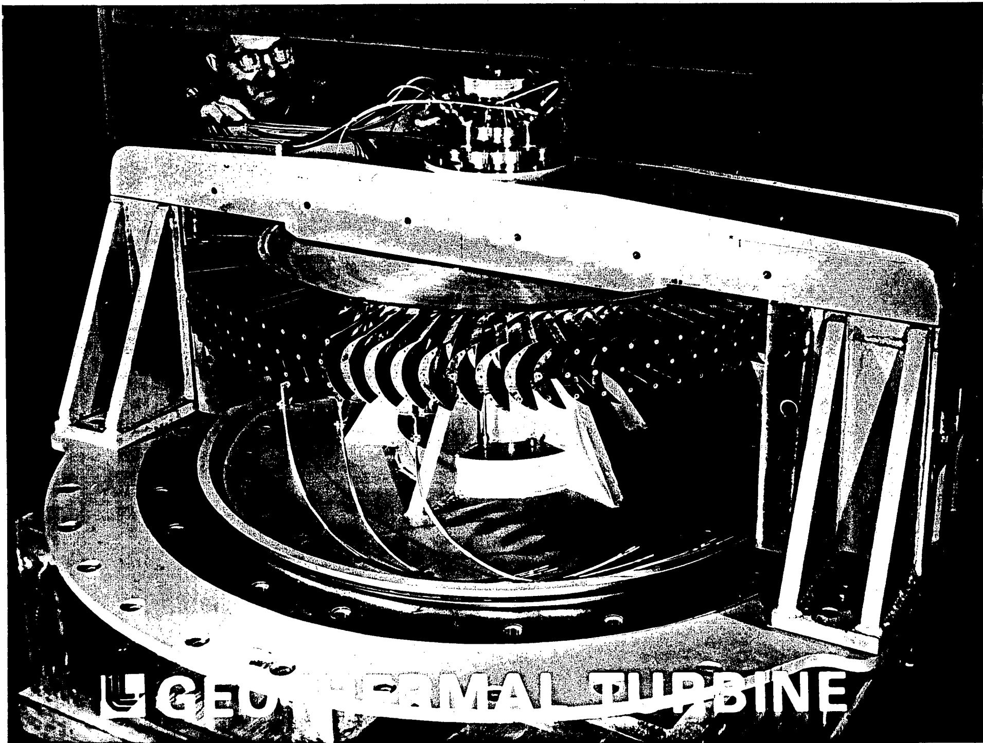
FIGURE 4-15. ASSEMBLY OF ROTOR INTO STATOR
