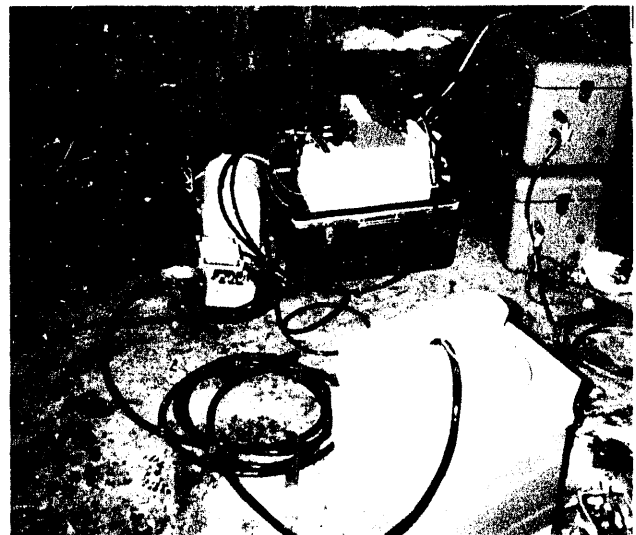
Figure 3. Remote seismometer vault at Pinedale. The Guralp sensor is in the foreground, enclosed in Styrofoam for thermal insulation, and the white box against the wall in the center is the digitizer. The fiber-optic cable interface, batteries, and connector cables are also shown.
