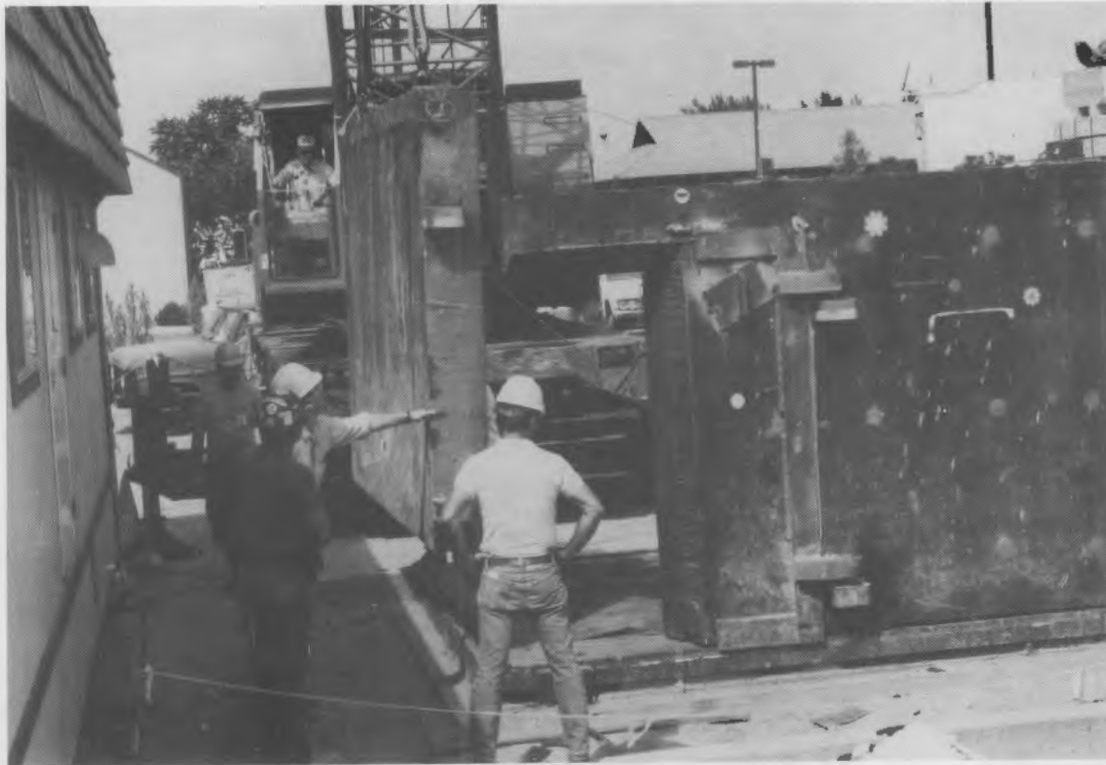
FIGURE 8. The Assembly of the Walls of the Utah Shielded Room
