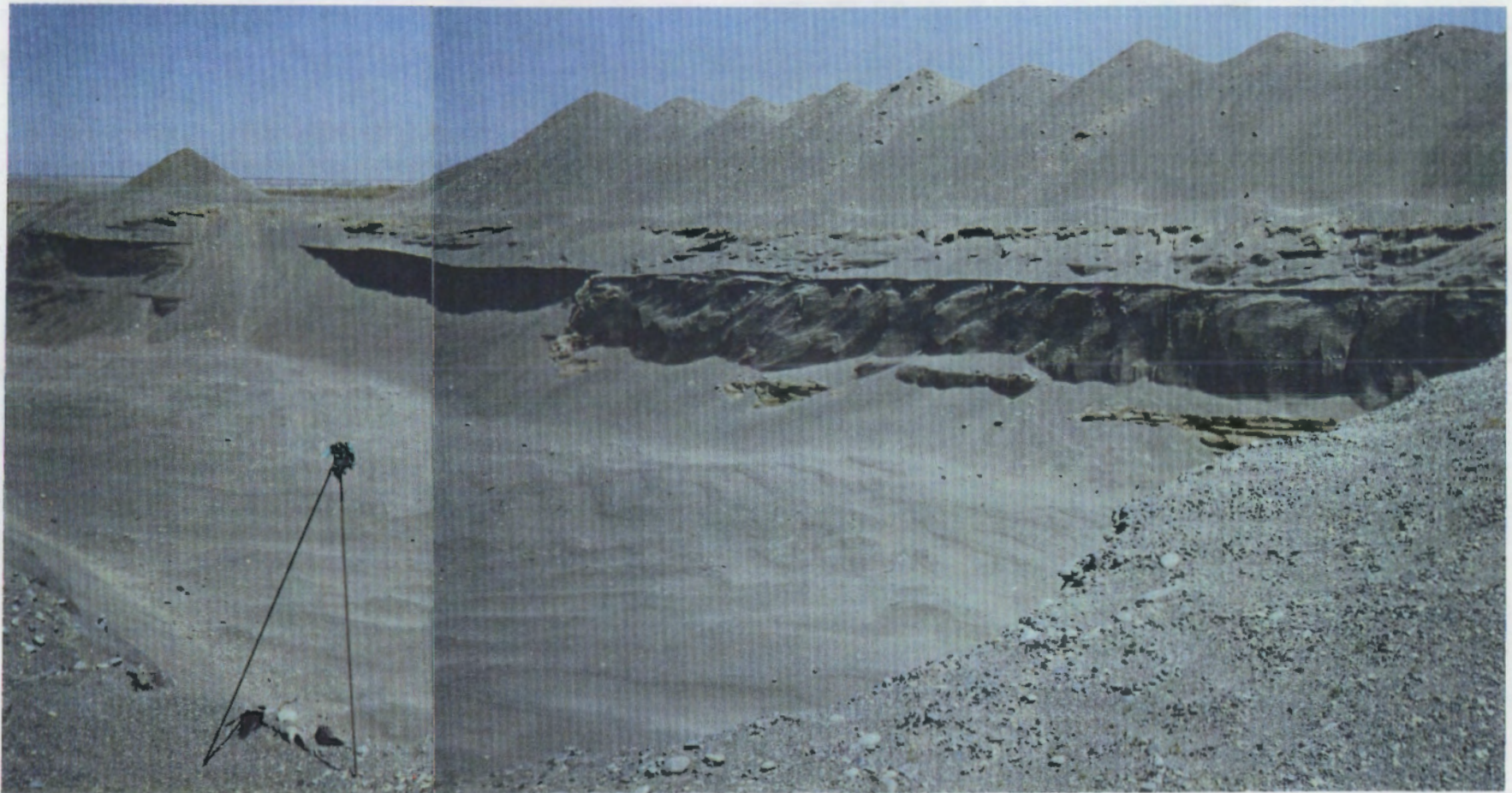
FIGURE 5. Large Trench Excavation at the Solid Waste Landfill. Spoil piles form a row of "hills" around the trench. The trench is excavated to a depth of 18 to 20 ft. The trench walls display distinct horizontal layers.
