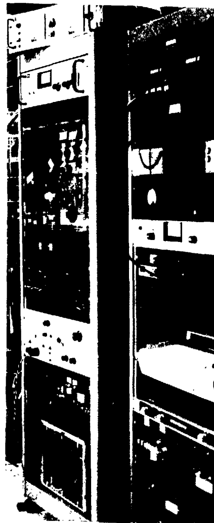
Fig. 2. Relay racks for operating LEE.
