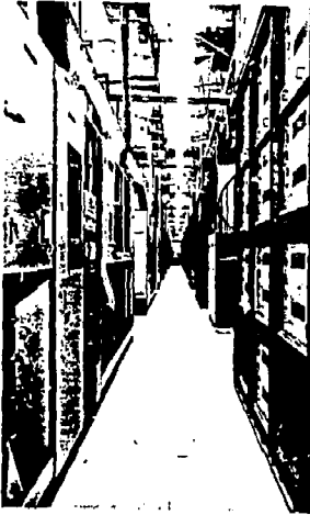
Figure 13 ATA Power Conditioning Area
