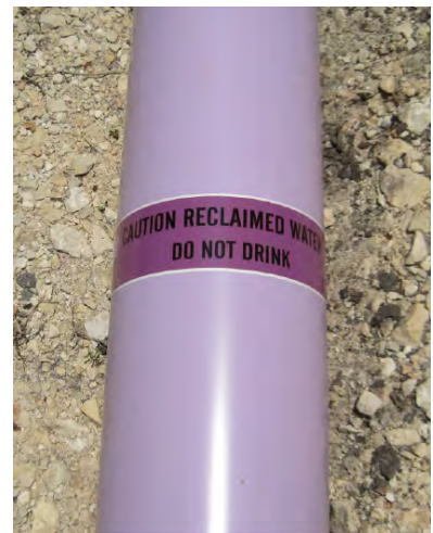
Figure 10.1 Purple tape with integral label wrapped around pipe
