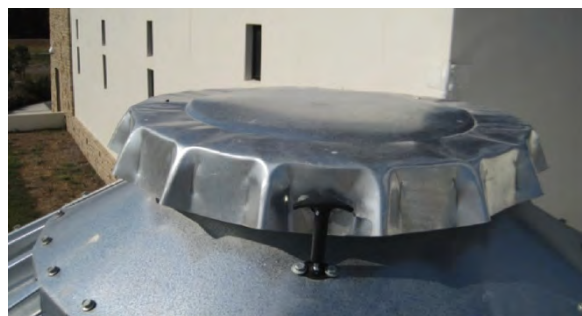
Figure 9.10 Round tank access port with locking lid
