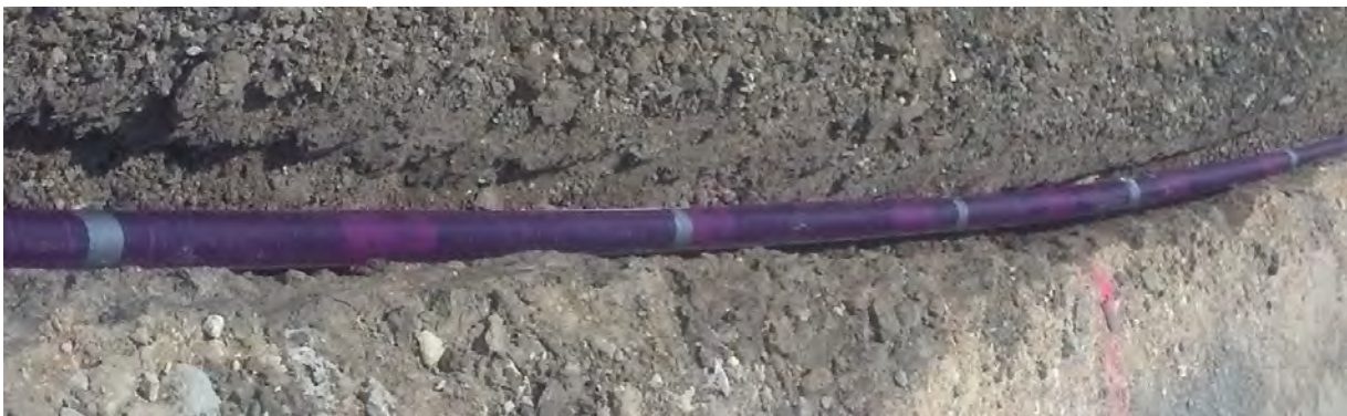
Figure 10.4 Color-coded purple label run lengthwise along top of pipe and taped firmly to pipe at regular intervals
