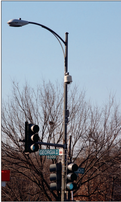
1.24 Streetlight surveillance camera and antenna in Washington D.C. Photograph taken by Jim Kuhn and shared via Creative Commons Attribution 2.0 Generic license.
