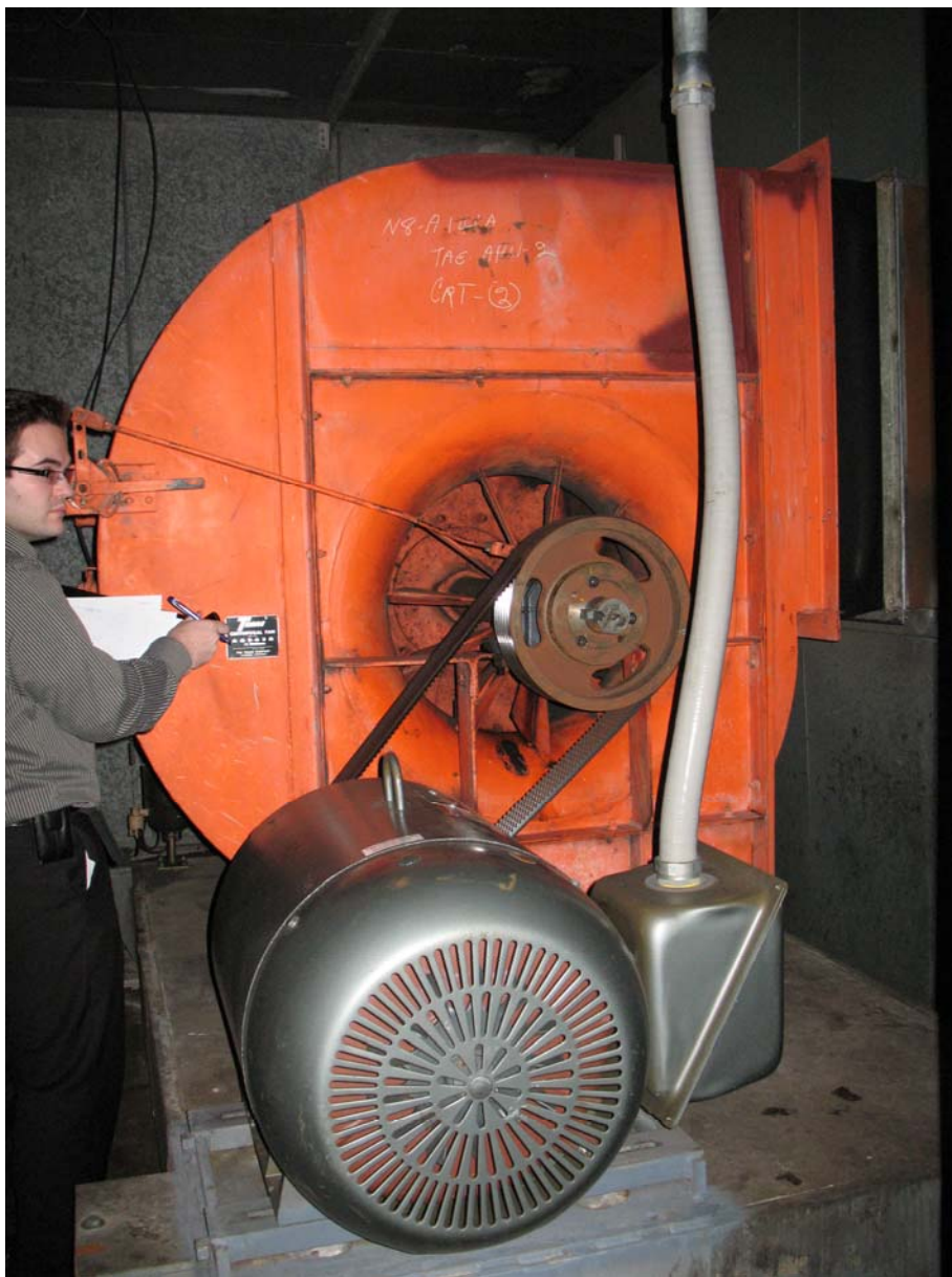
Photo 1: Joseph Blake, GSA Assistant Property Manager, collecting nameplate data from AHU-2 during FEMP audit site visit, December 2009.
