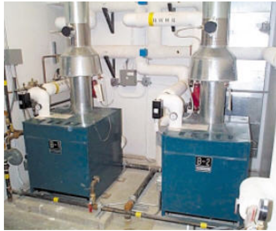
Figure 7. Exhaust Dampers Installed
