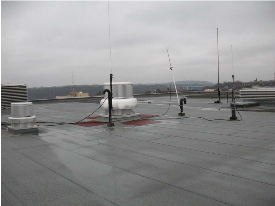
Photo 2: Roof area with potential for solar panel installation, December 2009.
