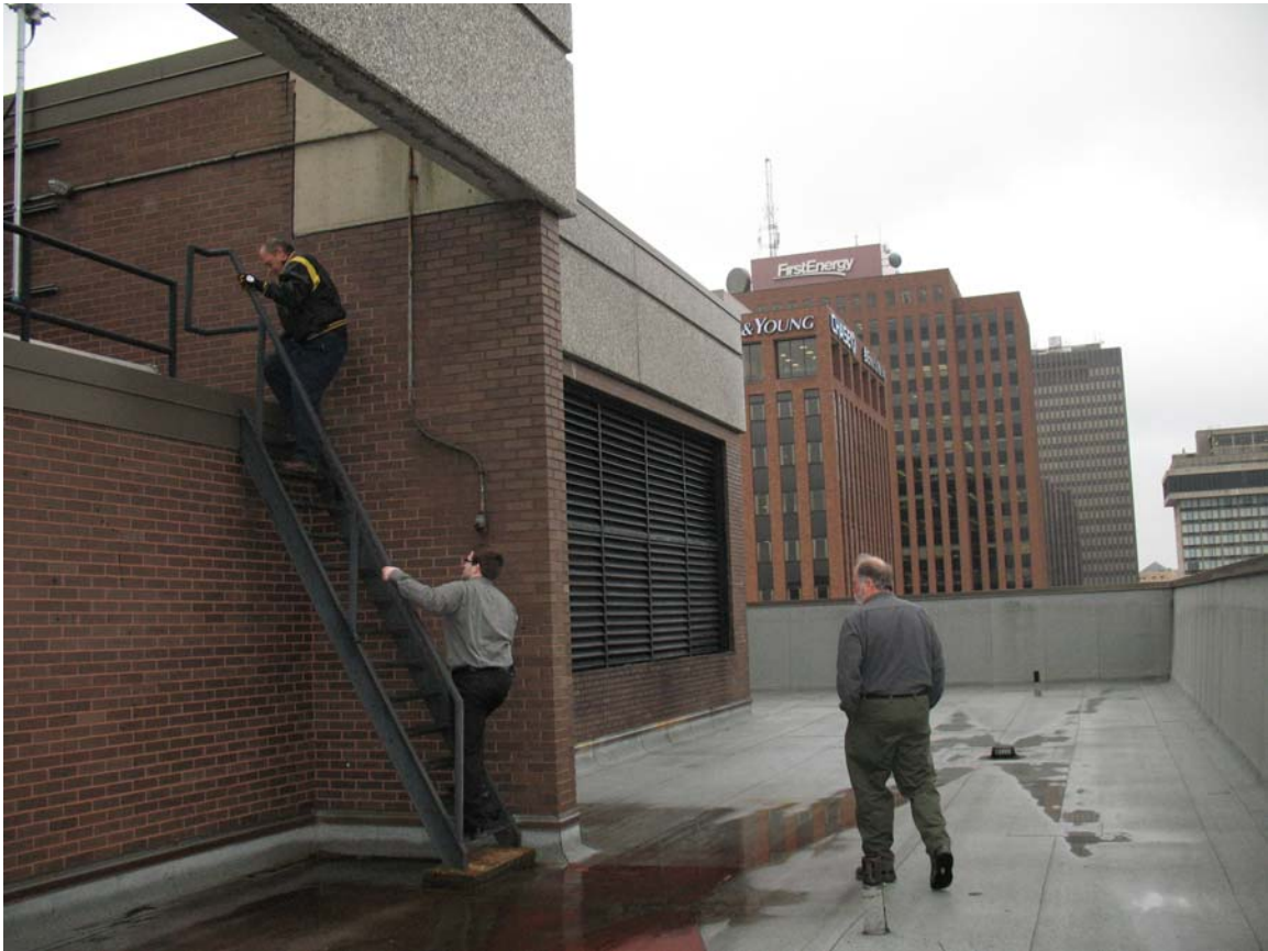
Photo 3: Harry Smith, maintenance mechanic with CMC & Maintenance, Inc.; Joseph Blake, GSA Assistant Property Manager; and Jim Arends, Redhorse Corporation CEM; climbing to collect data on rooftop BAC unit during FEMP audit site visit, December 2009.
