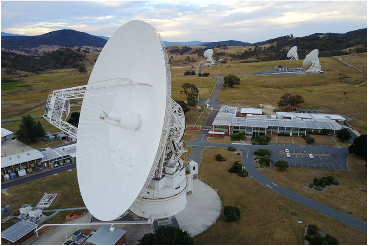
FIG. 3. Image of the Canberra Deep Space Communication Complex (CDSCC). The 70 m telescope (DSS-43) is shown in the foreground and the three 34 m beam waveguide antennas (DSS-34, DSS-35, and DSS-36) are shown in the background. Image credit: CDSCC a .
