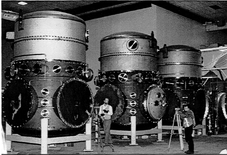
Figure 8. Photograph of surveyors measuring the locations of test mass chambers inside the corner station at the Hanford observatory. (December, 1997)
