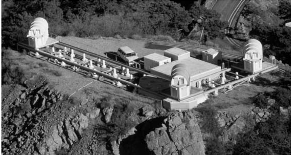
Figure 1. The IOTA interferometer on Mt Hopkins. All 3 telescopes are moveable, but shown here at their extreme end stations. Telescope A is left, telescope B is right, and telescope C is center. Both A and C move on the long (35 m) arm, and C moves on the short (15 m) arm.
