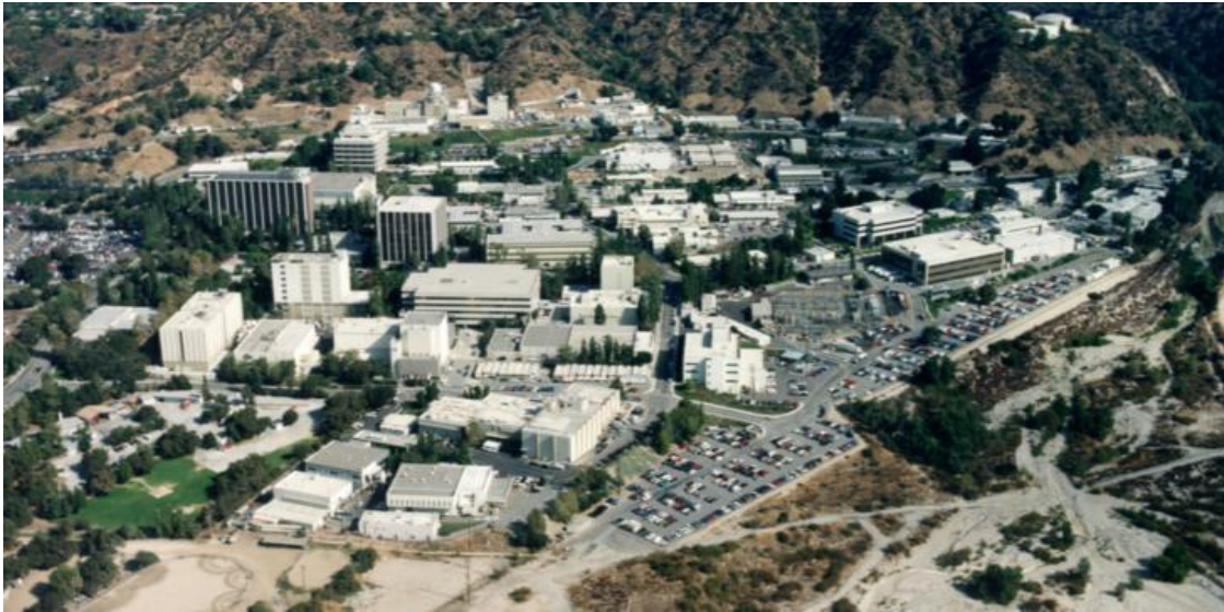
Fig. 2 - Aerial view of the NASA Jet Propulsion Laboratory showing the various types of structures on the campus and how density is similar to a cityscape ( Google Earth ).
