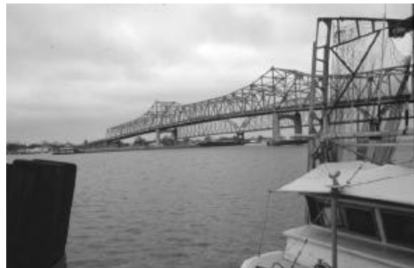
Figure 3.8. The bridge leaving Morgan City
