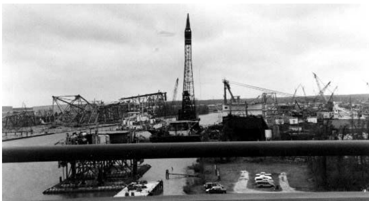
Figure 2.7. Fabrication yard in Amelia
