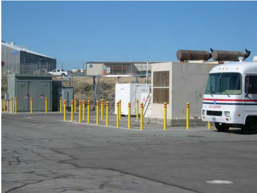
Site N3 area. Building 4889 was removed during the review period. The yellow bollards in the foreground indicate the former building footprint.
