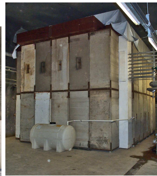
Figure 19: The NuMI Beam Hadron Absorber. The top Figure shows a schematic of the hadron absorber. The left bottom picture shows concrete block shielding around the downstream end of the decay pipe before the installation of the hadron absorber. The bottom right photograph shows the completed hadron absorber with the back wall of concrete blocks, and the steel roof blocks.
