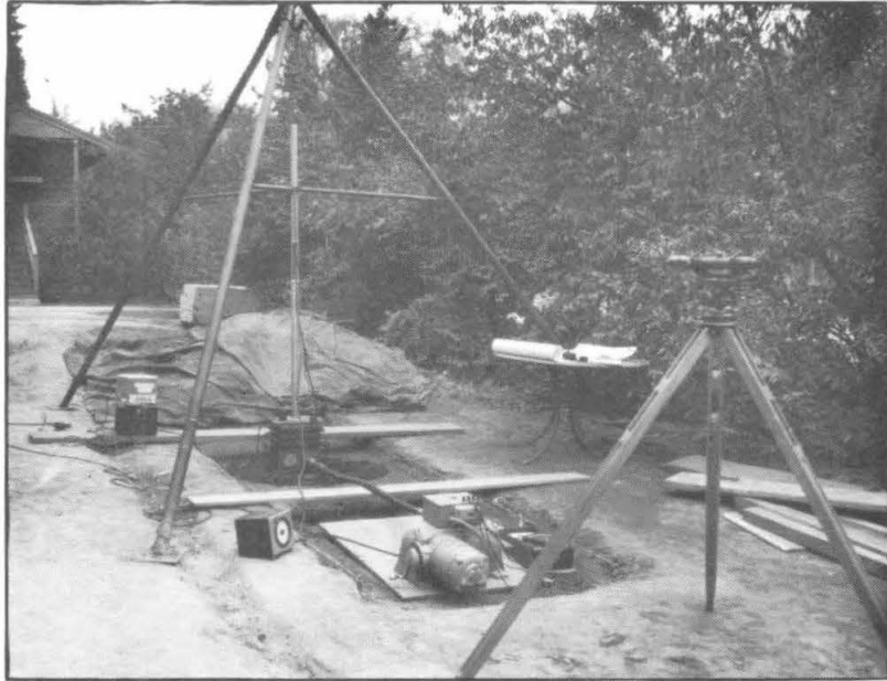
(A) Lazan Oscillator in position in Pit at C.I.T. before Vibration
