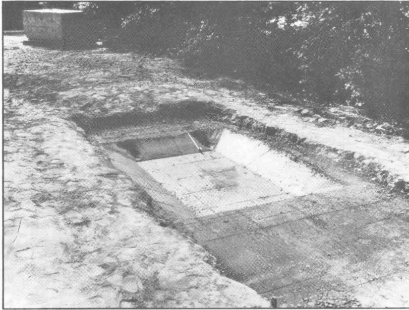
(A) Compacted area in Pit at C.I.T. after Tests V1 with Large Vibrator
