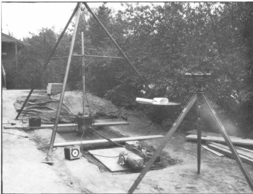
(B) Lazan Oscillator in position in Pit at C.I.T. after Vibration
