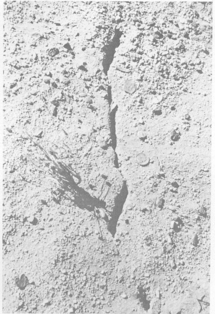
FIGURE 59. — Right-lateral displacement of about 2 cm on the Superstition Hills fault in sec. 23, R. 12 E., T. 14 S. Diameter of coin is 1.7 cm. Photograph taken April 22, 1968; note that crack has filled in since time of probable formation on April 9.
