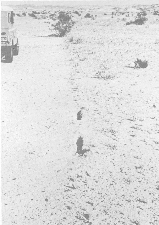
FIGURE 62. — Small collapse pits, alined vegetation, and variation in abundance of vegetation along the Superstition Hills fault in SW \frac{1}{4} sec. 9, T. 14 S., R. 12 E. New hairline cracks follow the alined features but are largely obscured by windblown sand and silt. Photograph taken May 14, 1968.
