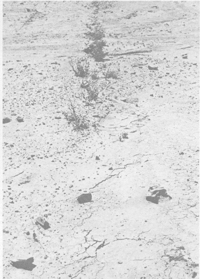
FIGURE 61.—New en echelon cracks of right-lateral habit following the line of desert plants that marks the Superstition Hills fault in NW \frac{1}{4} sec. 26, T. 13 S., R. 11 E. The larger plants are about 1 foot high. Photograph taken May 13, 1968.
