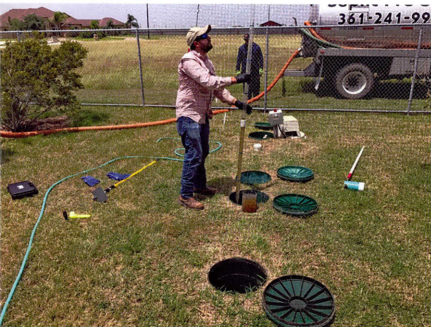
above: Septic System Inspection (Source: Ryan Gerlich, Texas A&M AgriLife Extension)
