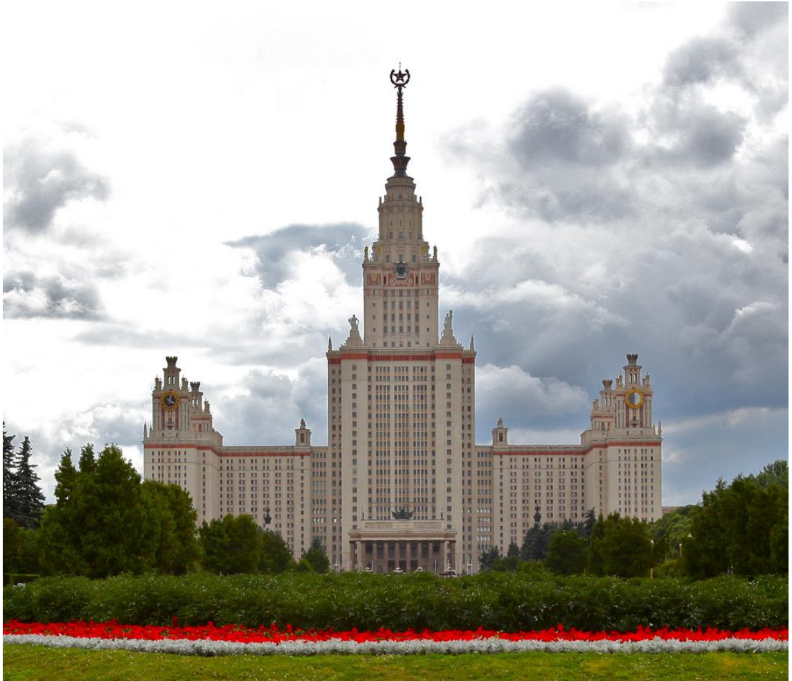
Figure 3. Main building of the MGU (Moskovskii gosudarstvennyi universitet im. Lomonosova). Constructed between 1949 and 1953, the building forms one of the seven Stalinist vysotki and is an excellent example of that era's 'wedding-cake' architectural style. Photograph, 'Moscow State University' © Steve Jurvetson, 2009, https://www.flickr.com/photos/jurvetson/5562359204/ (licensed under Creative Commons, CC BY Attribution 2.0, https://creativecommons.org/licenses/by/2.0/legalcode ).
