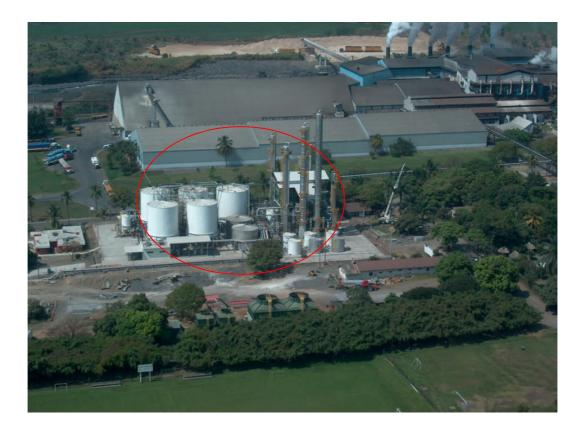
*Source*: Espinoza (2011). The fermentation units are located to the left of the photo, while the distillation towers are located towards the centre of the photo; the dehydration unit is not visible.
