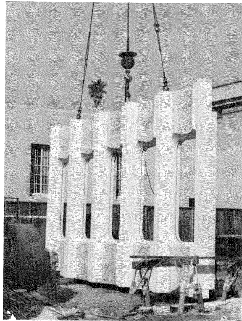
Fig. AV-7. ONE OF THE PRECAST CONCRETE WINDOW WALL PANELS.
