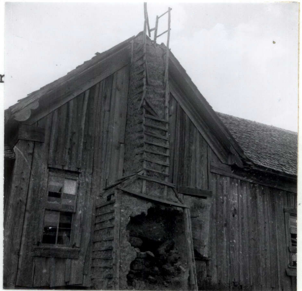
Fig. 21.--Mud-and-stick chimney in cabin about sixty-five years old.
