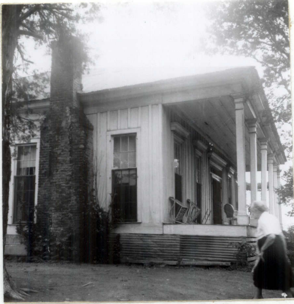
Fig. 16.--Williamson house, showing chimney.
