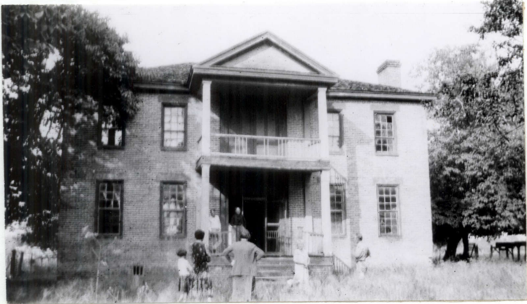
Fig. 33.--Oak Grove, before repairs
