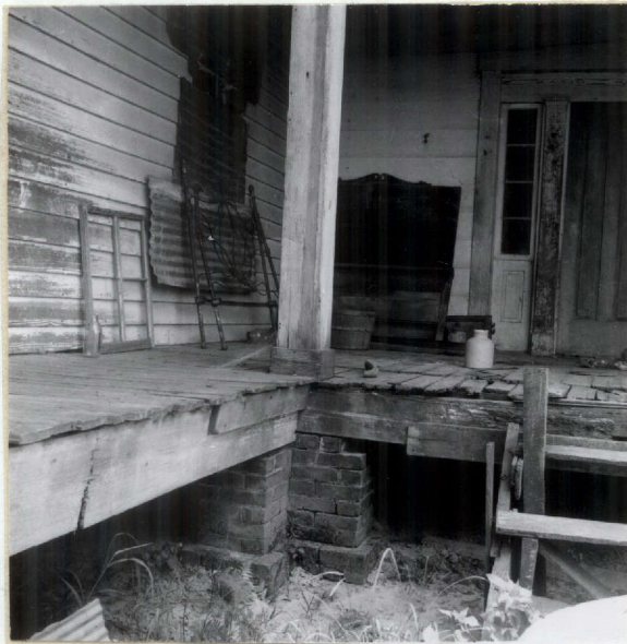
Fig. 14.--Right-angled brick piers, Bermuda Farm.
