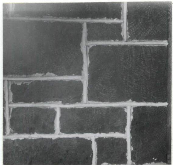
Fig. 19.--Detail of stonework, Henderson house, showing texture of pick marks.
