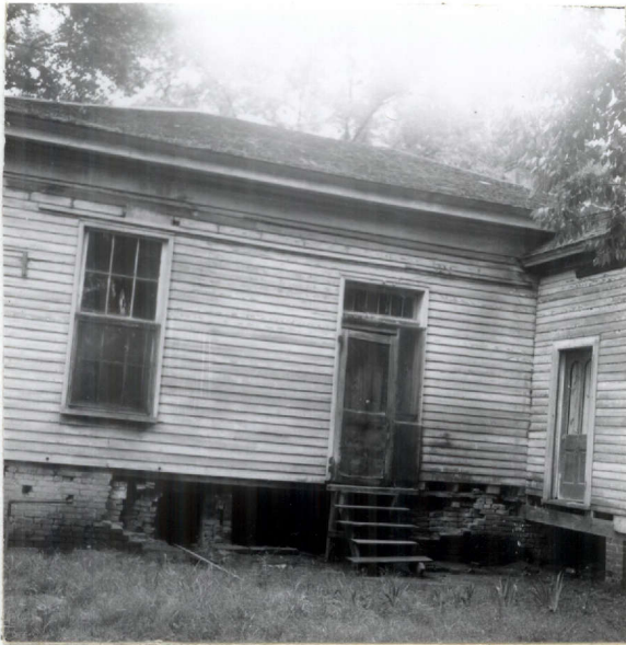
Fig. 15.--Henrich house, showing remains of foundation.
