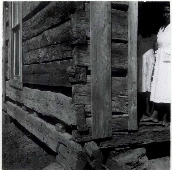
Fig. 3.--Mortise and tenon joints, Williams house.
