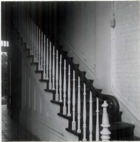
Fig. 8.--Walnut stair rail in Andrews house.
