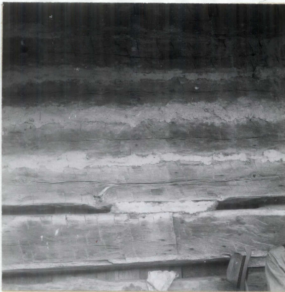
Fig. 22.--Mud-and-straw chinking in Williams house.
