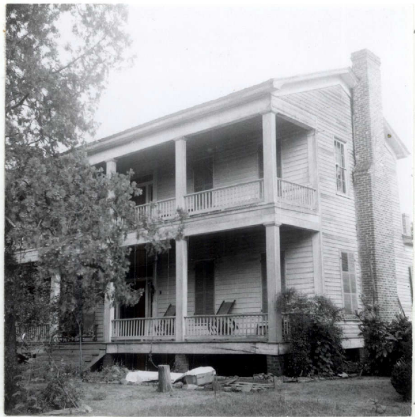
Fig. 17.--Locust Grove, showing chimney.
