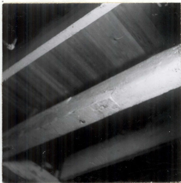
Fig. 5.--Spliced joint with oak peg, Bernstein house.
