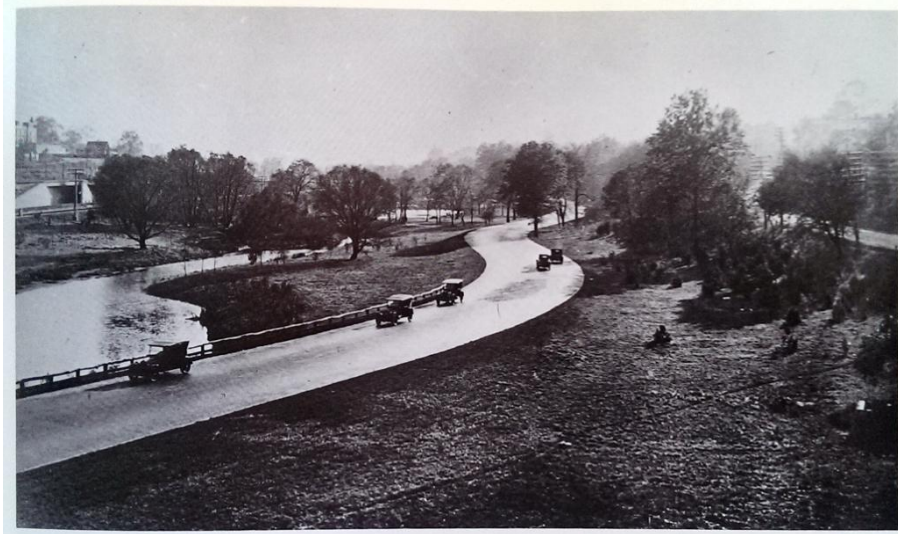
Figure 2.25: Gilmore D. Clarke, Bronx River Parkway, 1922, section near Woodlawn, NY, photograph, Newton Collection, Frances Loeb Library, Graduate School of Design, Harvard University, From The Machine Age , 95.
