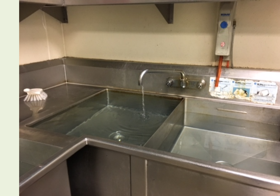
Figure 10. Three full wash basins of 165L each in the RDC back kitchen with faucet still running, no dishes being washed, and no staff attendants; approx. 500L of wasted water from this single occurrence.
