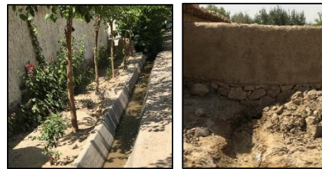
Photograph 10: Joiborho in Khatlon Province, Tajikistan. Left: Cement lined joibor running between road and household compound wall. Right: Joibor running from a watercourse under a household compound wall into their yard. Photos by author.
