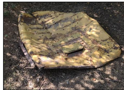
Photograph 8: An old car door that is used as a make-shift water gate in Khatlon Province, Tajikistan after the gate installed in the Soviet period went missing. Photo by author.
