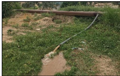
Photograph 6: Pump system drawing water from a tertiary canal to pipes that empty into intra-village watercourses in Khatlon Province, Tajikistan. The pump is operated and maintained by a local resident who took the job when no one else in the village felt qualified. Having studied physics in grade school made the transition easier, he explained, but otherwise he has learned everything related to the pump system on his own. Despite his care, leaks have sprung all along the pipes leading from the pump station into the village. A lack of funds has led to improvised solutions like red piece of metal pictured, which is successfully blocking a leak. Photos by author.
