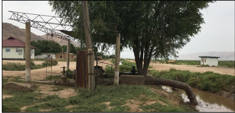
Photograph 6: Pump system drawing water from a tertiary canal to pipes that empty into intra-village watercourses in Khatlon Province, Tajikistan. The pump is operated and maintained by a local resident who took the job when no one else in the village felt qualified. Having studied physics in grade school made the transition easier, he explained, but otherwise he has learned everything related to the pump system on his own. Despite his care, leaks have sprung all along the pipes leading from the pump station into the village. A lack of funds has led to improvised solutions like red piece of metal pictured, which is successfully blocking a leak. Photos by author.
