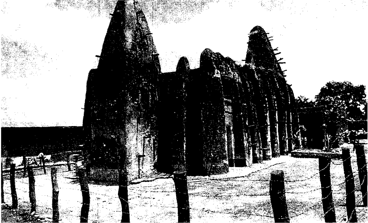
Fig. 3. Sudanic-style, timber, and clay mosque at Manluwe, Upper West Region. The preservation of mosques in northern Ghana is a of the Ghana Museums and Monuments Board (photograph courtesy of C.R. DeCorse). [end of page 101]
