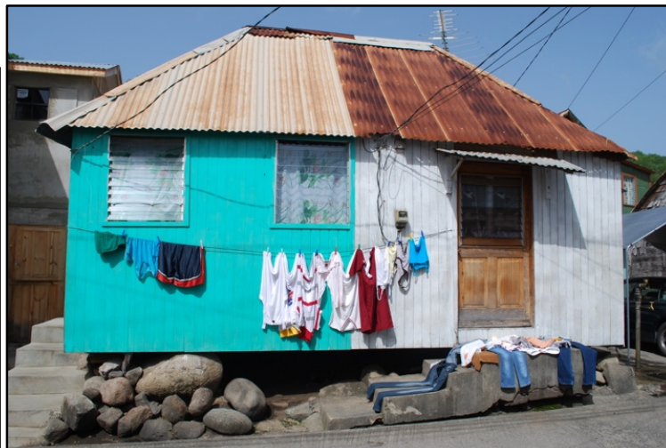
Figure 5.15: Vernacular housing style identified in Dublanc, Dominica that relies on unmortared piles of stone to buttress the side of the structure (photo by Z. Beier).
