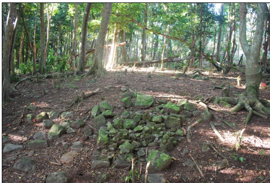
Figure 5.28: The north wall of "barrack 2" in CG-2 with entryway (photo by Z. Beier).
