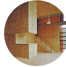
Figure 23. They approach the interior stair and glass doors.
