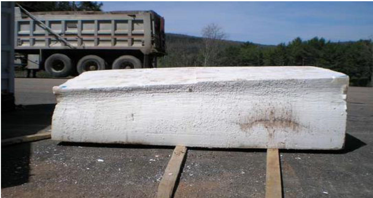
Figure 29: Removed Geofoam Variable Deformation (GEB, 2008)
