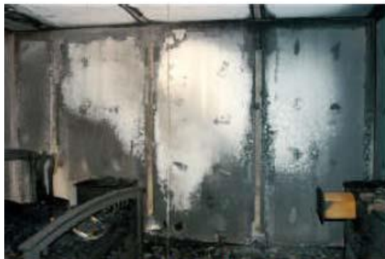
Figure 6. View to W wall of cell 3 showing a large, clean-burn "V-pattern"
