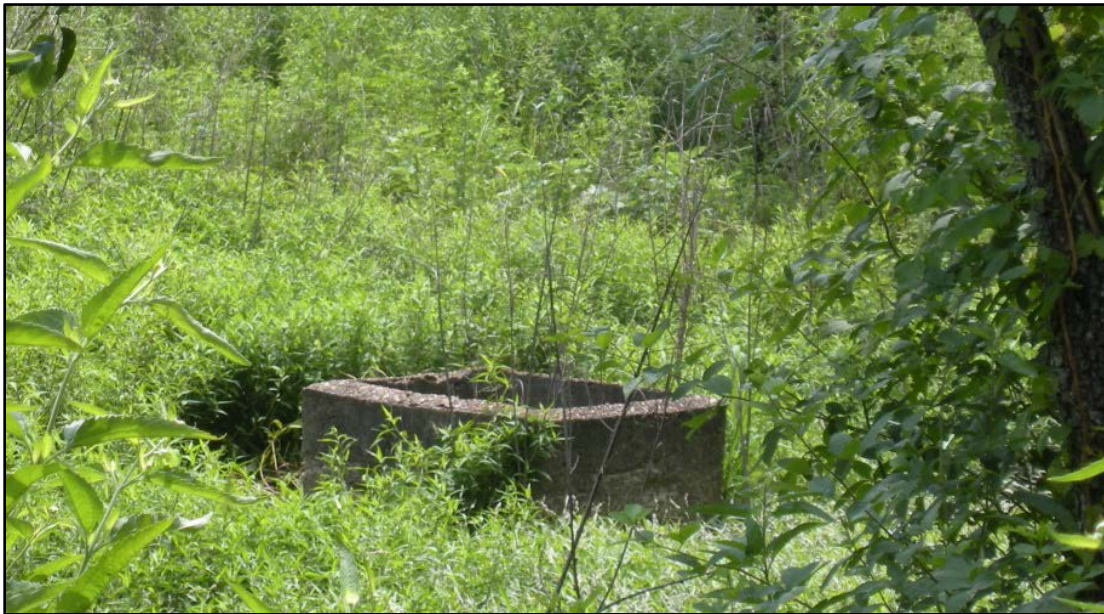
Figure 5.17 Spring box located north of the Taylor household, built by Benjamin Jackson, facing northeast (S. Loftus).
