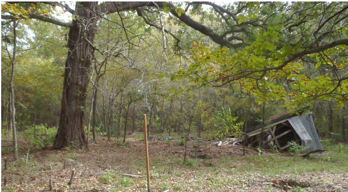
Figure 5.4: Overview of collapsed structure at the Davis Site (41AN188), facing east. The shovel handle is in the location of the Feature 2, the well (S. Loftus).
