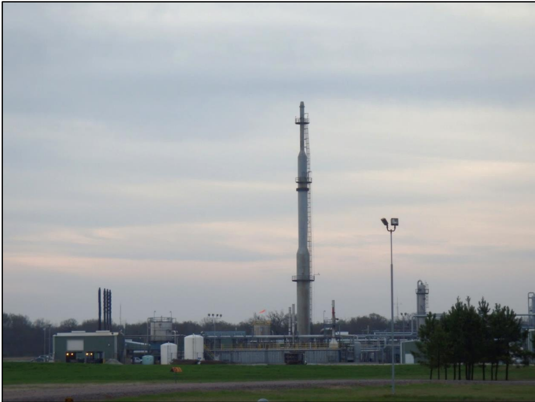
Figure 3.17: Substation located south of the Benjamin Jackson Plantation (S. Loftus)
