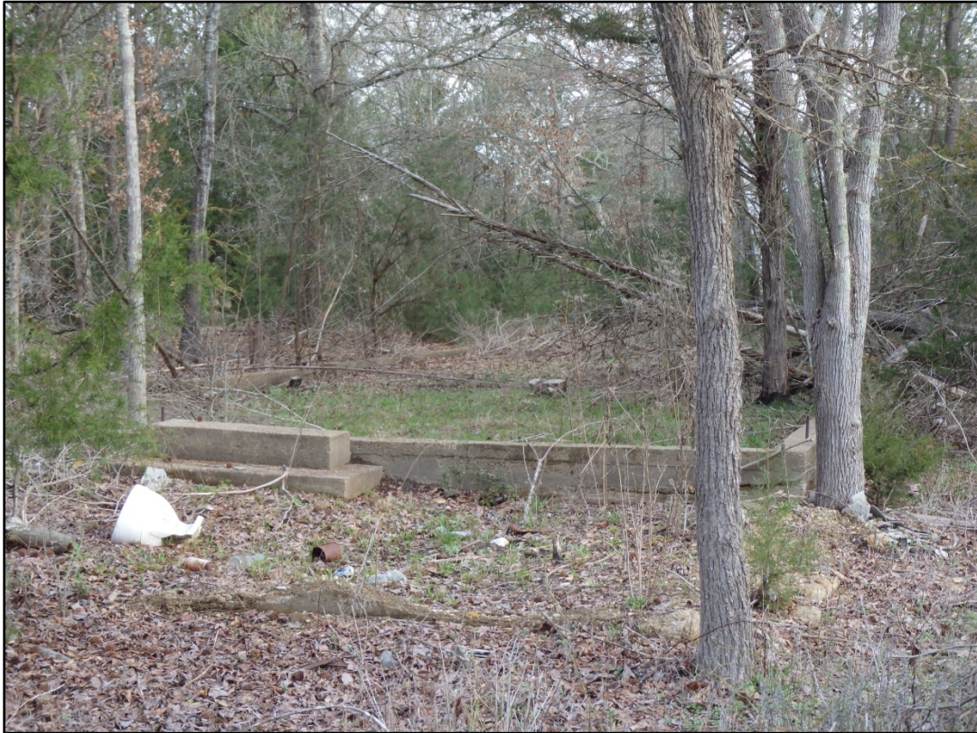
Figure 3.14: Bethel School Foundation (S. Loftus)
