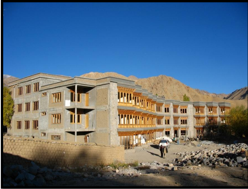
14. Druk Hotel under construction in 2008. Photo by author.
