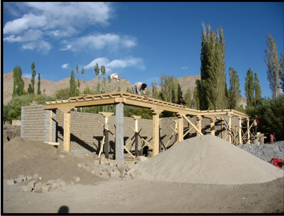
36. The Namgyal Sister's restaurant under construction. Photo by author.
