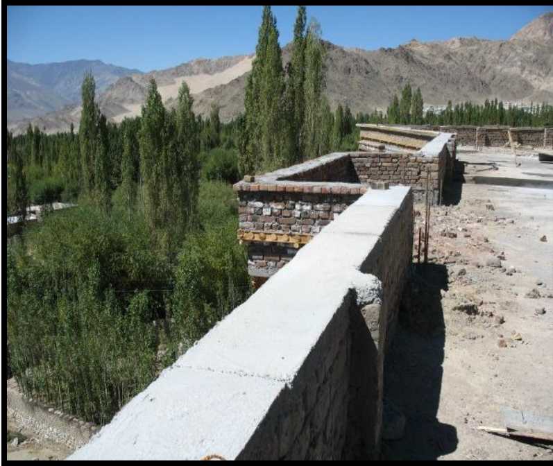
33. Above and below: The Dragon Hotel roof had brick on the outside; mud brick, brick, and stone on the inside. Photos by author.
