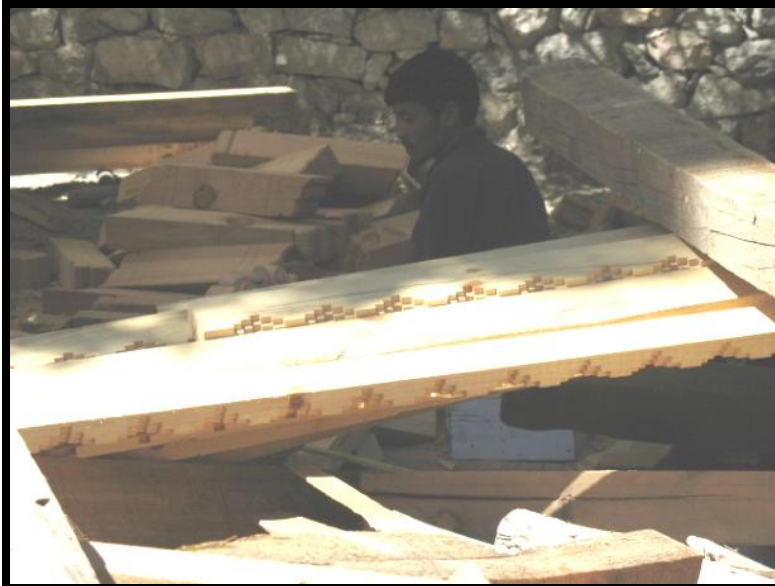
13. A man carves decorative exterior adornments from a pile of lumber at the Hotel Dragon construction site. Photo by author.
