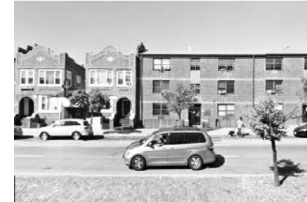
HOWARD AVENUE , 1988 5 Buildings, 3-Stories Tall
