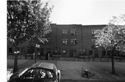
HOWARD AVENUE-PARK PLACE , 1994 8 Buildings, 3-Stories Tall
