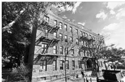
SUTTER AVENUE-UNION STREET , 1994 3 Buildings, 4- and 6-Stories Tall
