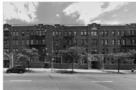
TAPSCOTT STREET REHAB , 1986 8 Buildings, 4-Stories Tall
